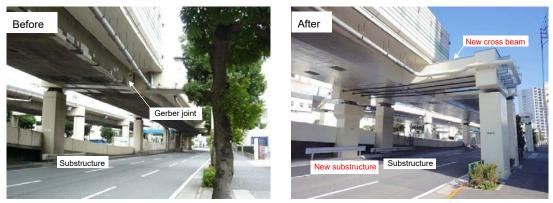
Photo 6. Gerber joints separated with new substructure
