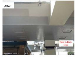
Photo 5. Gerber joints made continuous
